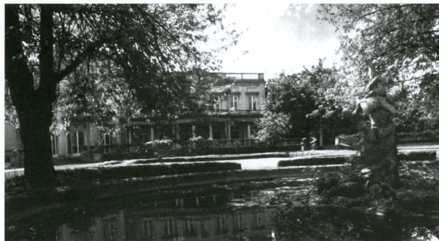
Froebel College, one of the four colleges that make up the Institute's West London campus and currently the location for a six month site-specific event by Forster and Heighes exploring the ethics of building.
